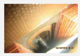
Figure 1: Loose nut on PA core leg phase 1
