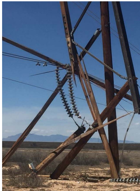
Figure 9 Other Fire Damaged Structures
