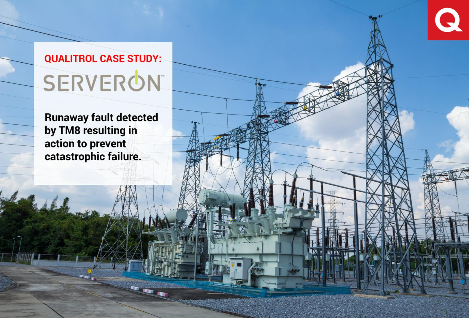
On August 28th, 2016 a Serveron DGA was being used to monitor a 3-phase, 1100 MVA, 345 kV GSU.
